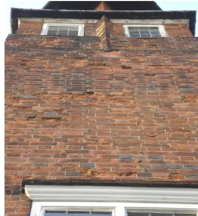
It is also interesting to note that the original mortar would have been black, and indeed one can still see black mortar in protected parts of the walls and elsewhere around Brentham, for example under the eaves.
