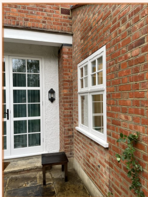
Matching new and old brickwork and careful positioning of where the new wall meets the old
